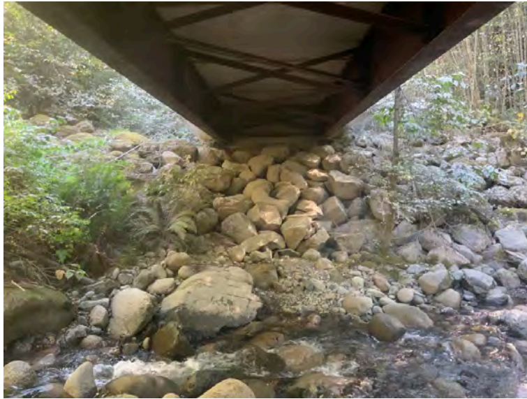
Left Bank Abutment when facing downstream
