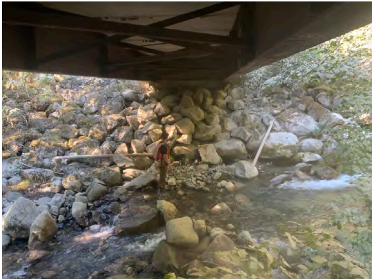
Right Bank Abutment when facing downstream
