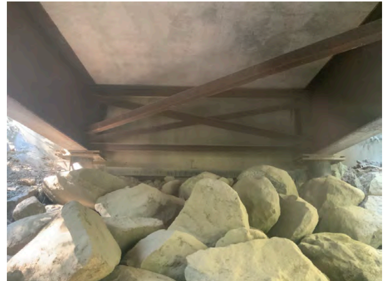
Right Bank Abutment when facing downstream
