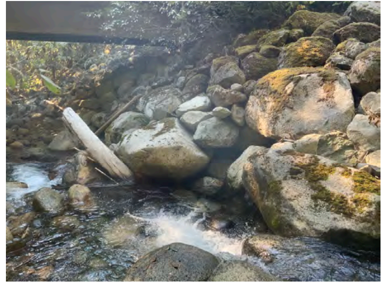
Right Bank Abutment when facing downstream
