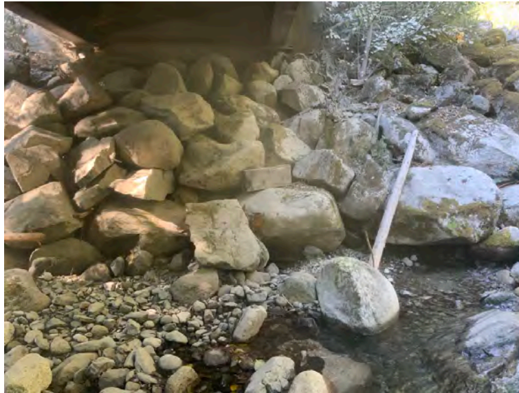
Right Bank Abutment when facing downstream
