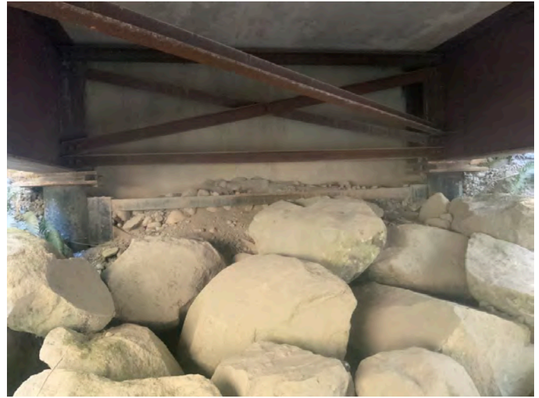
Left Bank Abutment when facing downstream
